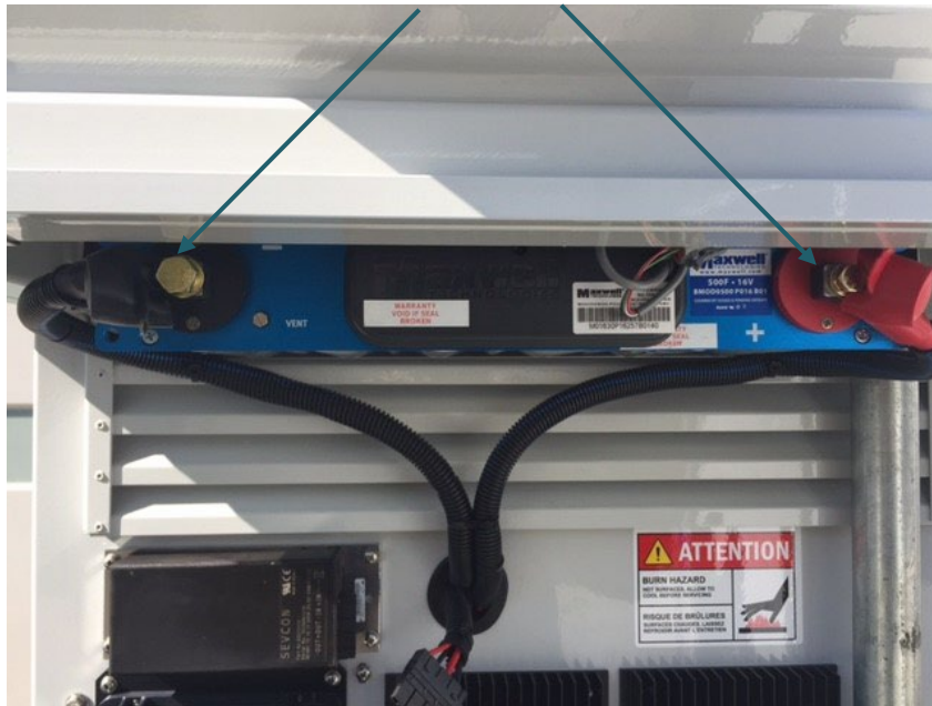
Figure 16 – Supercapacitor Terminals
