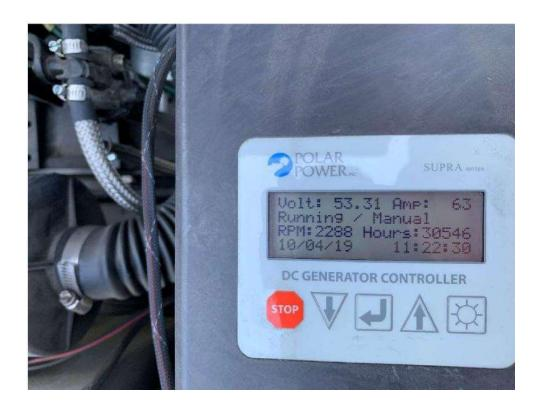
Results from past 4 years were taken as part of this study at this site with a continuous generator run time of over 30,546 hours and continuing. There were no failures from any critical components in the generator like the alternator, controller, engine, radiator, or the modems. There are no apparent issues that might indicate that an engine overhaul or replacement may be necessary.
