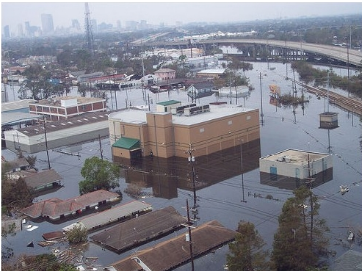
Fig. 5.77. Aerial view of New Orleans Sprint long-distance switch taken on September 1, 2005 [28]
