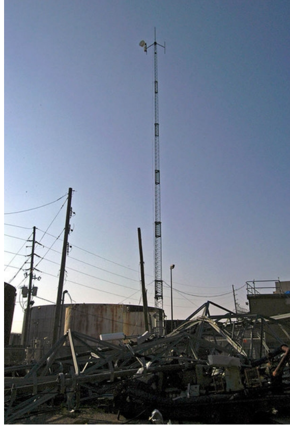
Fig. 9.1. Fallen antenna in Jefferson Parish sheriff office building [45]
