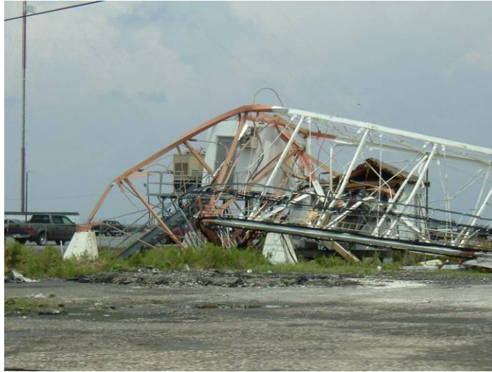
Fig. 6.37. Fallen Tower in Leeville, LA [36]
