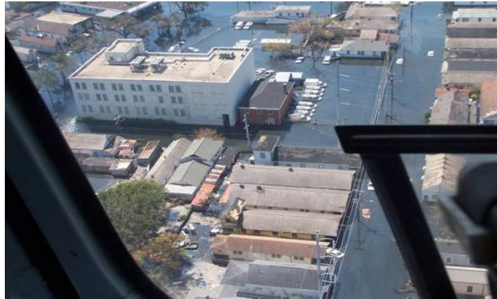
Fig. 5.64. Aerial view of Franklin CO [20]
