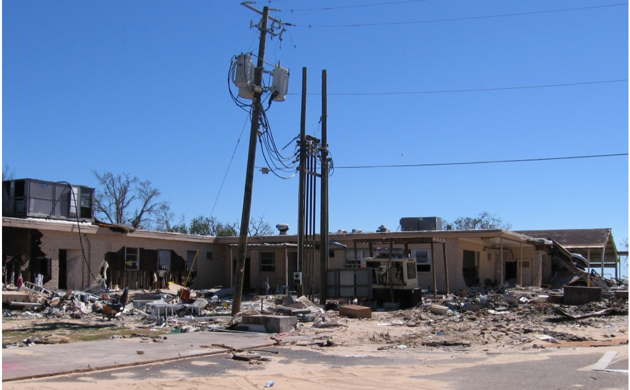
Fig. 9.6. Destroyed nursing home in Pass Christian, MS
