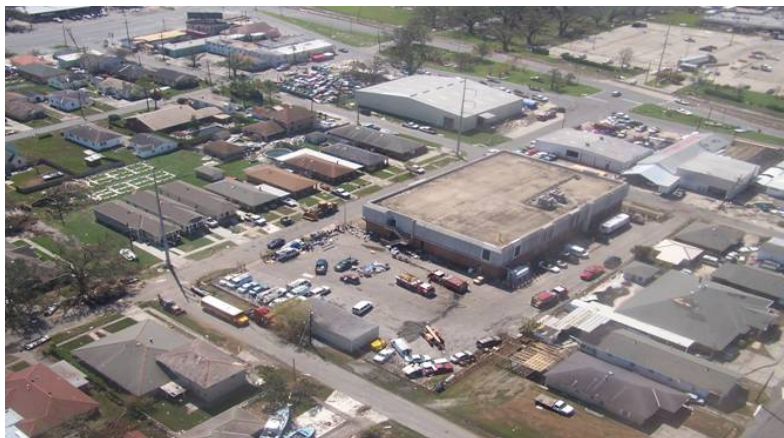
Fig. 5.66. Aerial view of Chalmette CO [20]
