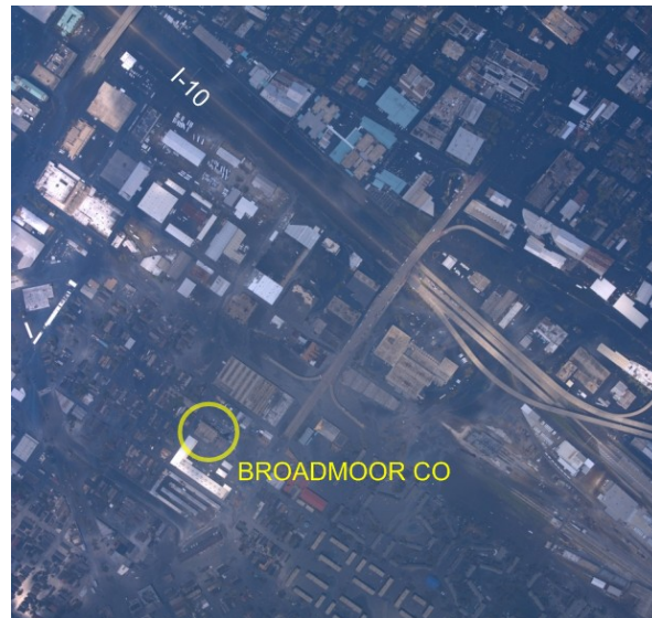
Fig. 5.59. Aerial view of Broadmoor CO, August 31, 2005 [6]
