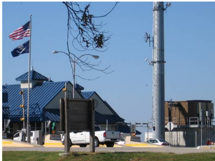
Fig. 6.59. Cell site next to Lake Pontchartrain Causeway Toll
