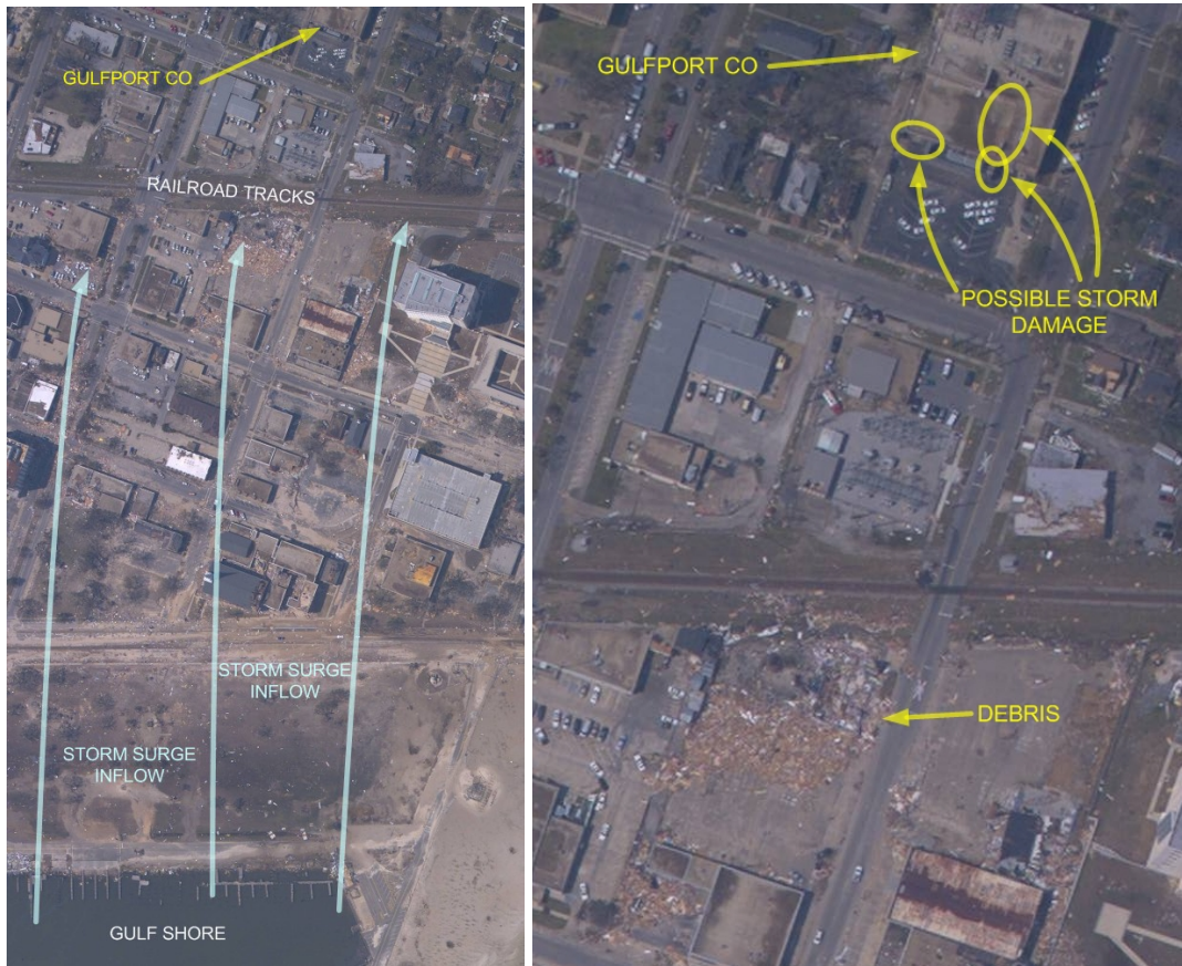
Fig. 5.23. Aerial view of Gulfport CO, August 30, 2005 [6]
