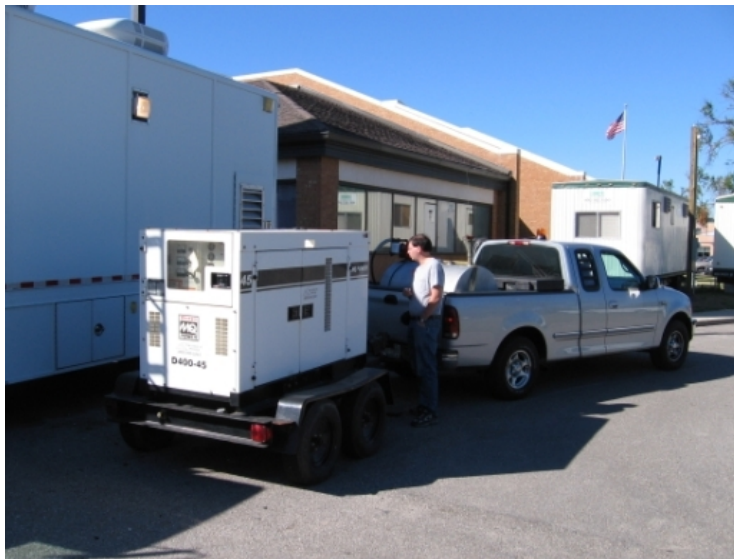
Fig. 2.19. Refueling the genset that provides power to a Biloxi cell site
