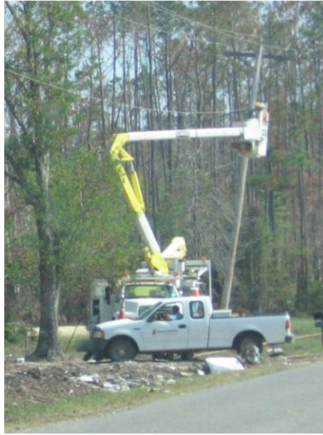
Fig. 3.12. PSTN outside plant being repaired
