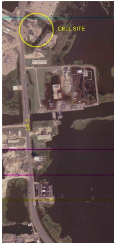
Fig. 6.38. Aerial view of the cell site with the fallen tower in Leeville, LA [10]
