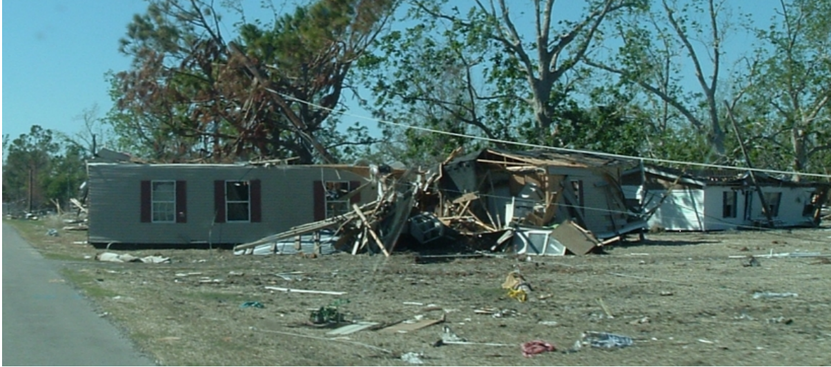
Fig. 3.4. Total destruction on Highway 15, LA
