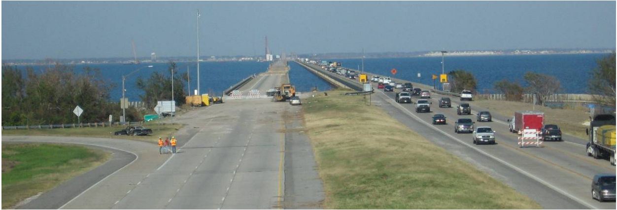
Fig. 1.2. I-10 bridge over Lake Pontchartrain
