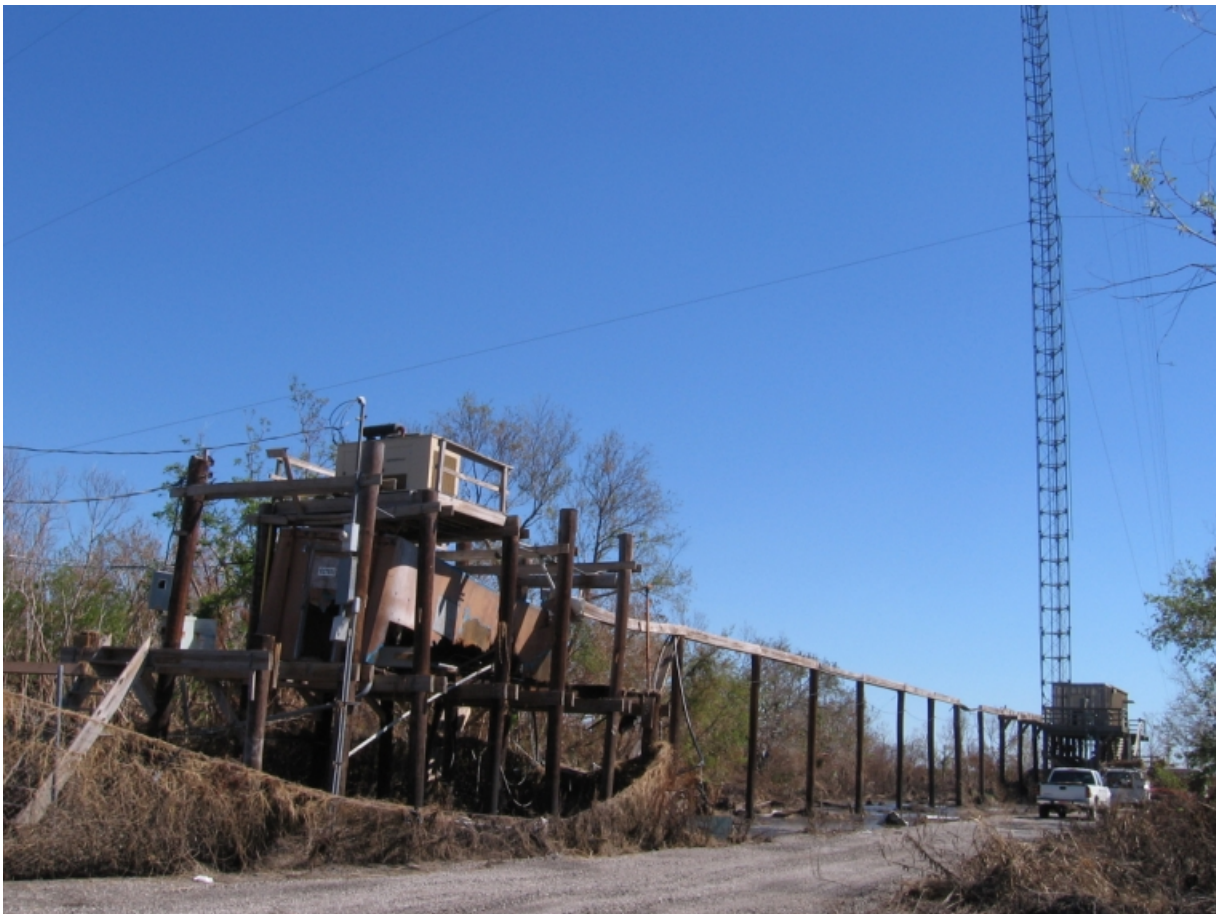
Fig. 7.1. KQLD-FM Radio transmitter and tower in Delacroix, LA
