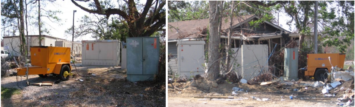
Fig. 5.85. Two views of a DLC system in Waveland, Bay St. Louis CO
