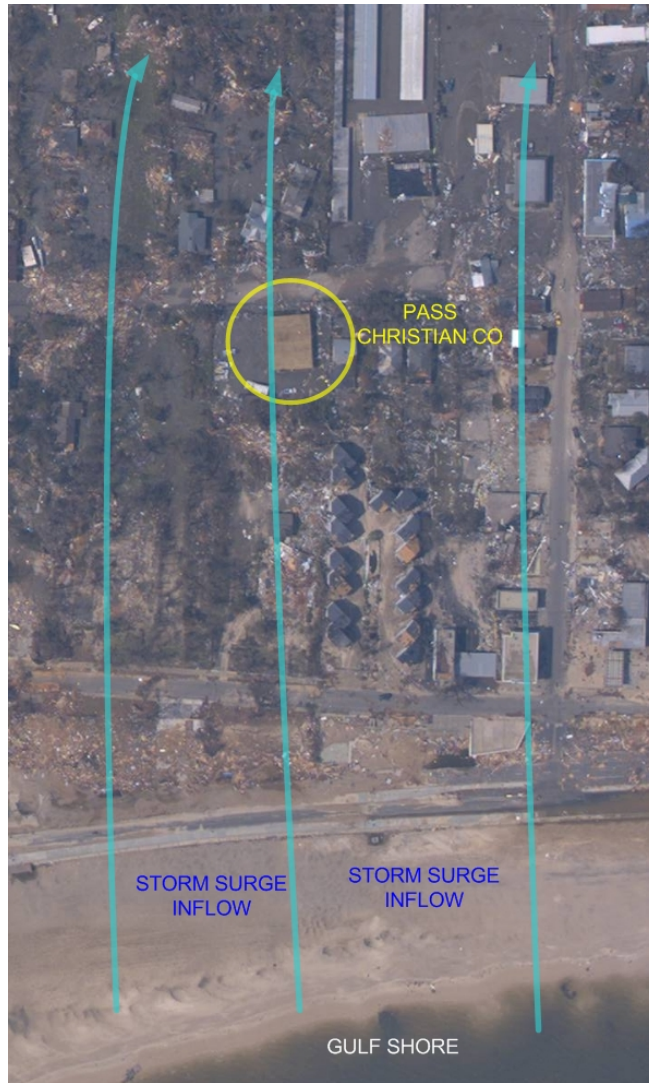
Fig. 5.31. Aerial view showing vulnerable location of Pass Christian CO, August 30, 2005 [6]
