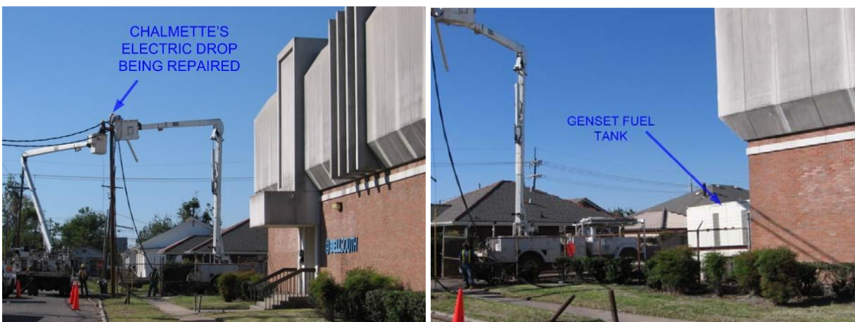
Fig. 5.67. Chalmette electric drop being repaired
