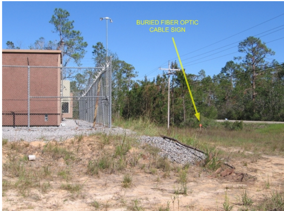
Fig. 5.83. Level3 transmission site showing its location on elevated terrain
