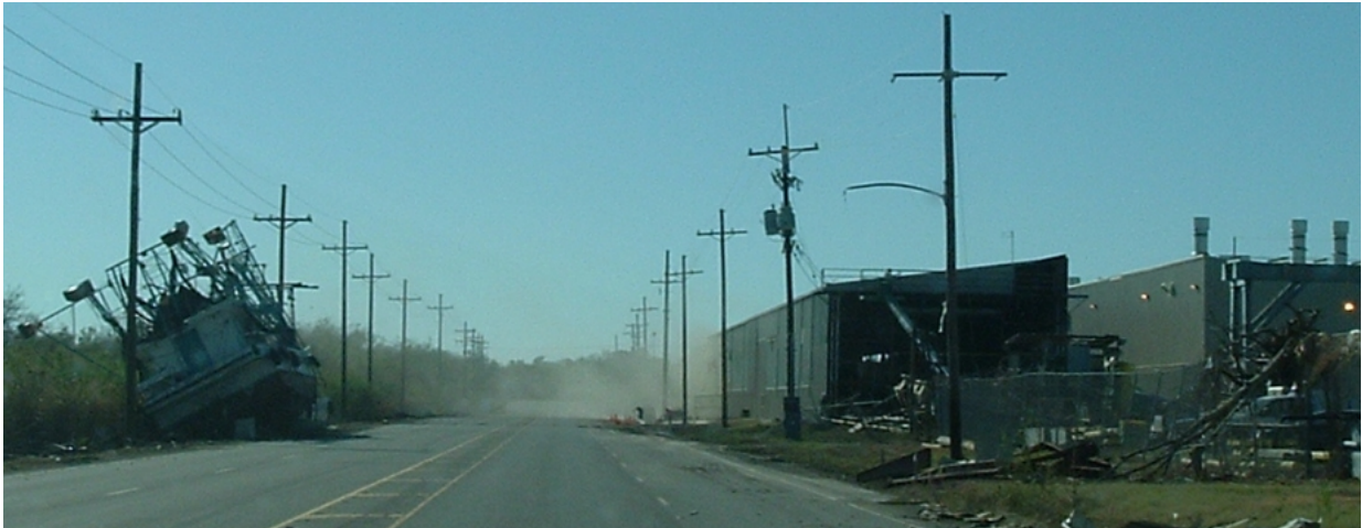
Fig. 3.17. Electrical and communication infrastructure in good condition on Route 90 northeast of New Orleans
