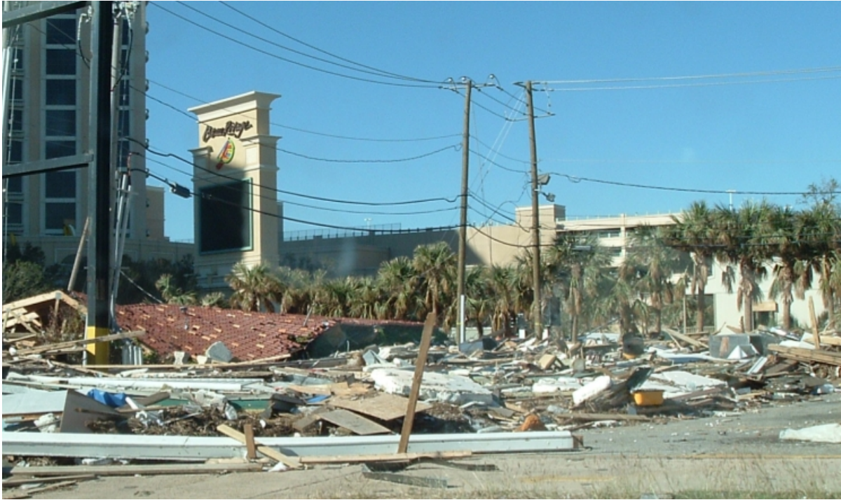
Fig. 3.8. Light damage to poles amid total destruction to buildings in Biloxi, MS
