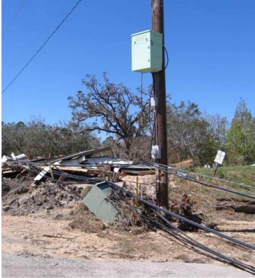
Fig. 7.11. Pole-mounted and pedestal-mounted CATV UPSs.
