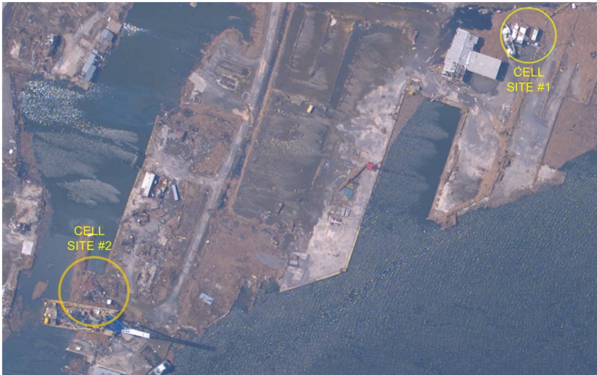
Fig. 6.9. Aerial view of destroyed cell sites in Venice, LA [6]
