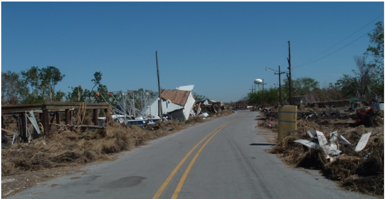
Fig. 3.11. Severe damage to construction but light damage to electrical and communication networks in Delacroix, LA
