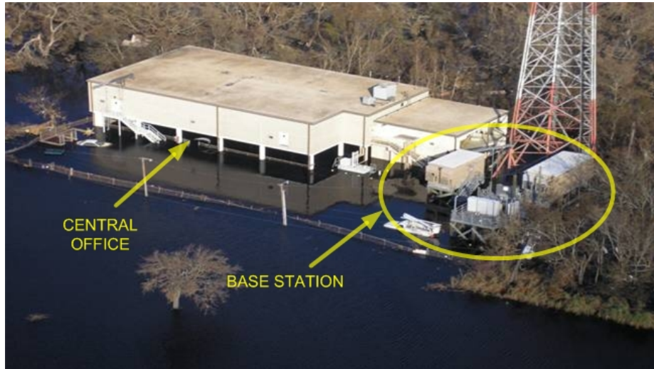
Fig. 6.14. BellSouth Buras CO showing the collocated cell site [20]
