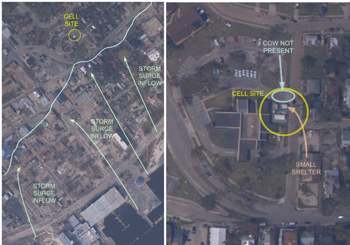
Fig. 6.31. Aerial pictures of cell site in Biloxi, August 30, 2005 [6]
