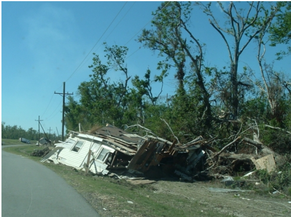
Fig. 3.9. Total destruction to houses but light damage to electrical infrastructure near Point A La Hache, LA
