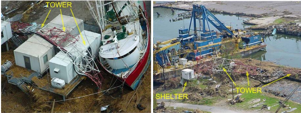
Fig. 6.8. Aerial view of destroyed cell sites in Venice, LA [34]
