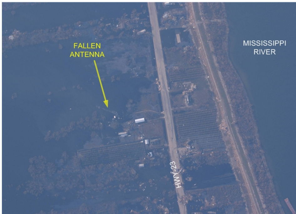
Fig. 6.13. Aerial view of destroyed cell site in Port Sulphur, LA September 3, 2005 [6]
