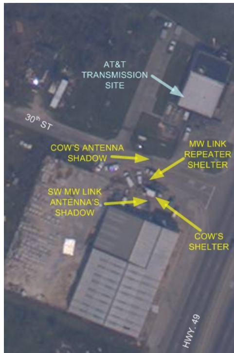
Fig. 6.64. Aerial shot of Sprint Nextel COW and emergency transmission repeater, September 4 th [6]
