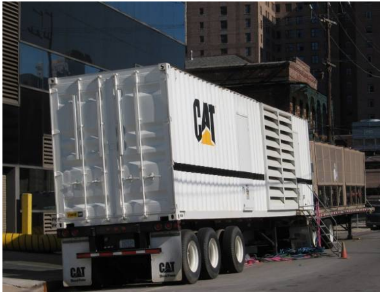
Fig. 2.18. Caterpillar portable power trailer
