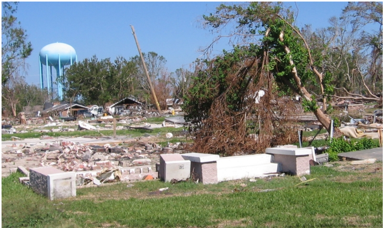
Fig. 3.1. Severe destruction in Biloxi, MS
