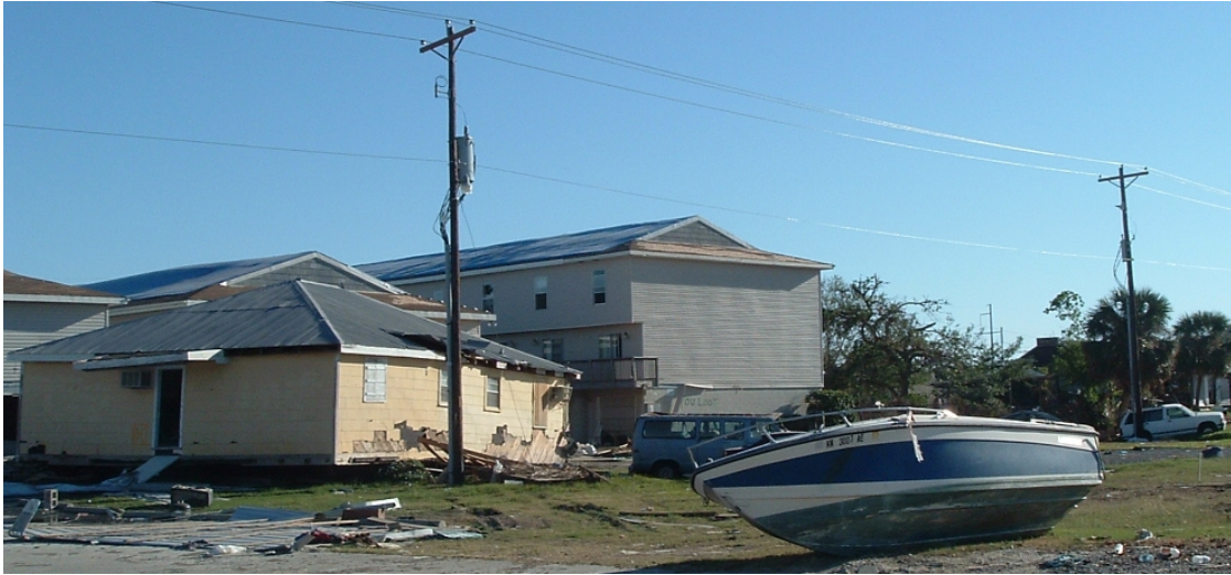
Fig. 3.16. House lifted from foundation, boat, and undamaged poles in Slidell, LA
