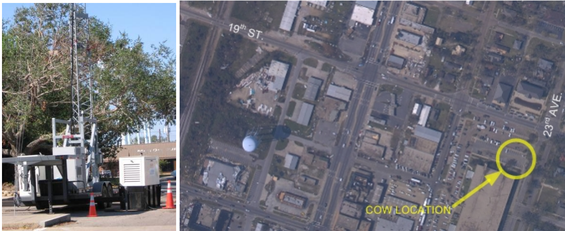
Fig. 6.65. (a) Left: COW in Gulfport, (b) Aerial picture taken on August 30 th of the area where the same COW was installed [6]
