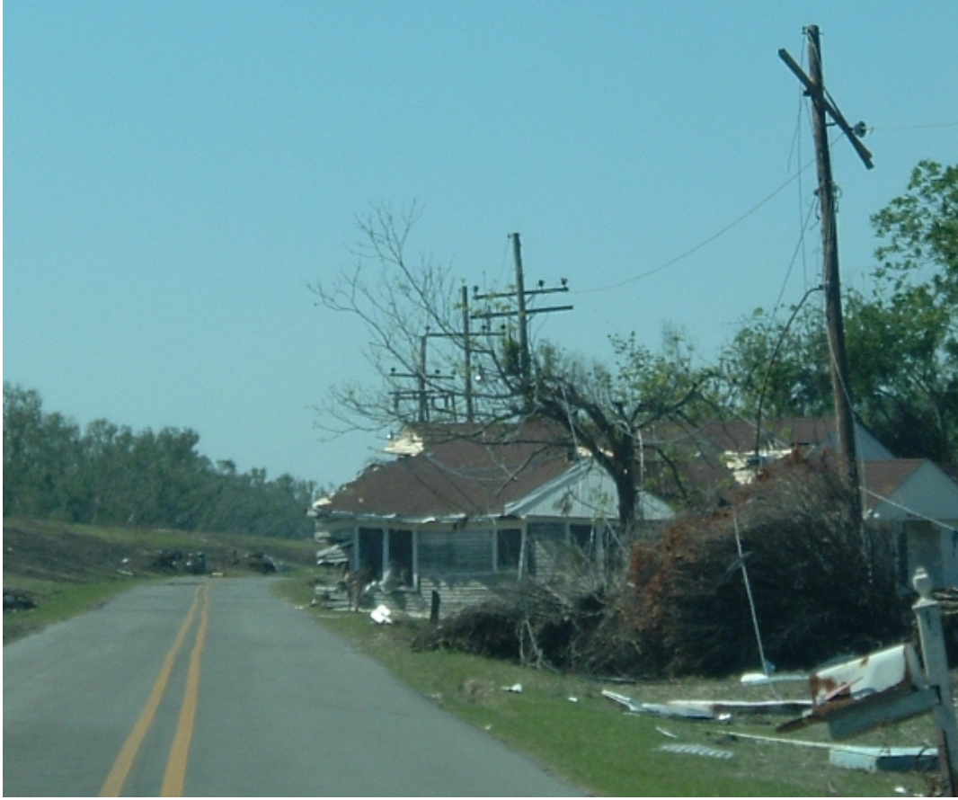
Fig. 3.14. Damaged pole and hanging wires on Highway 15, LA
