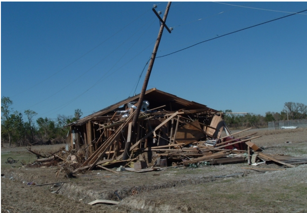
Fig. 3.13. House crashed on a pole on Highway 15, LA
