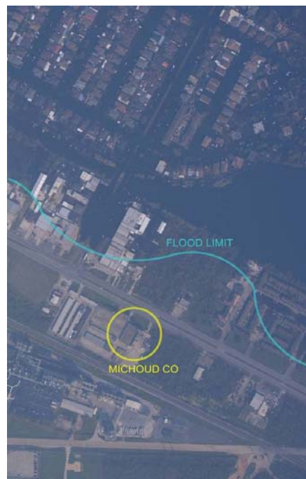
Fig. 5.69. Aerial view of Michoud CO, September 3, 2005 [6]
