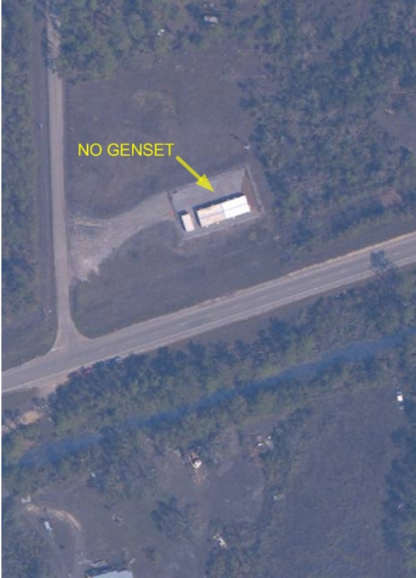
Fig. 5.82. Aerial view of Level3 transmission site, September 2, 2005 [6]
