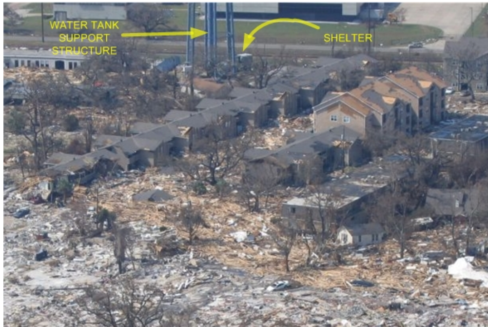
Fig. 6.22. Damage next to water tower cell site [9]
