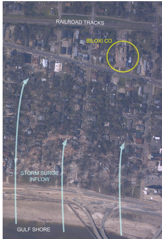
Fig. 5.26. Aerial view of Biloxi CO, August 30, 2005 [6]
