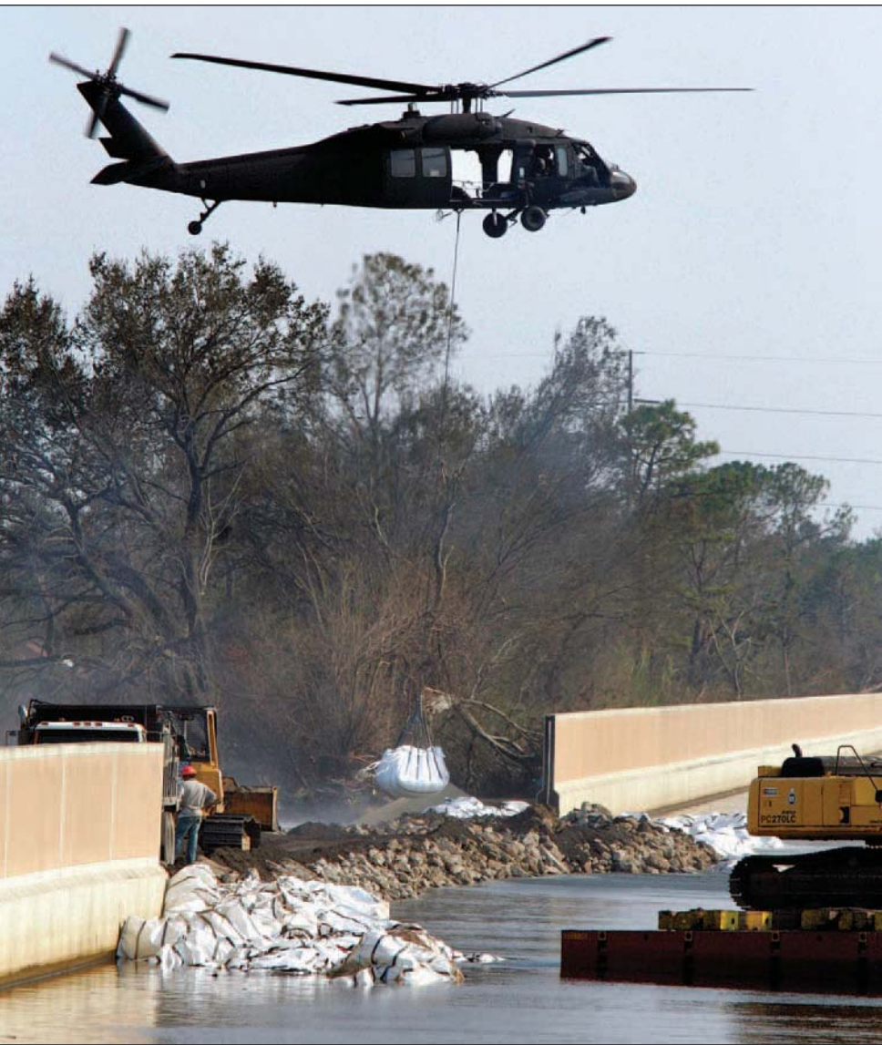
Plugging a breached floodwall, New Orleans
