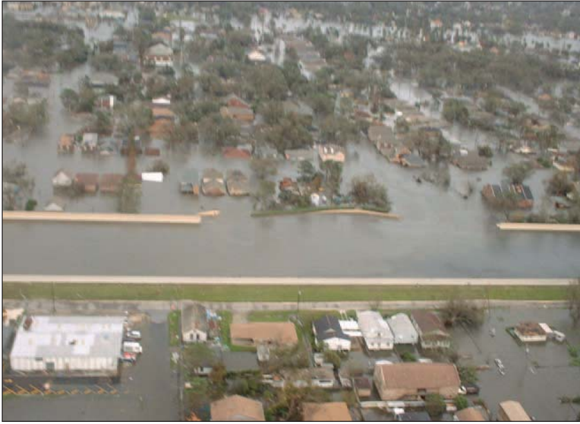
Breached floodwall, New Orleans Marty Bahamonde photo
