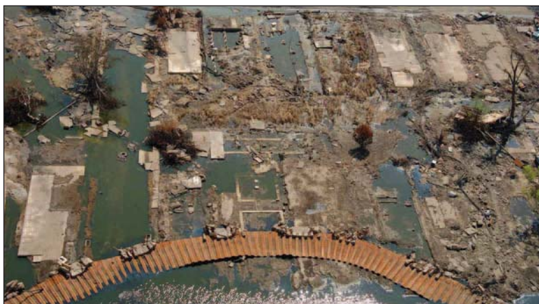
Ripped-out sheetpile with chunks of floodwall attached, New Orleans Louisiana National Guard photo
