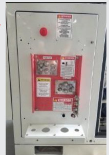
Electrical tie on
