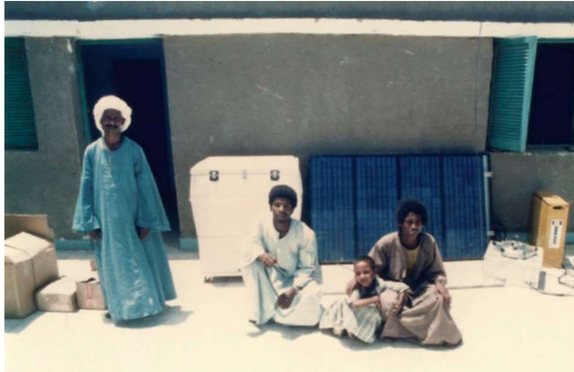
Our UN installation trip to Egypt in the 1980s The high cost of solar necessitated a secondary energy source, leading us to explore small wind generators.
